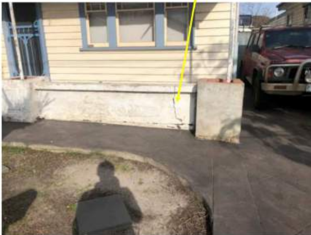
Subject crack dating back to 2014 – evidence of crack opening over time
