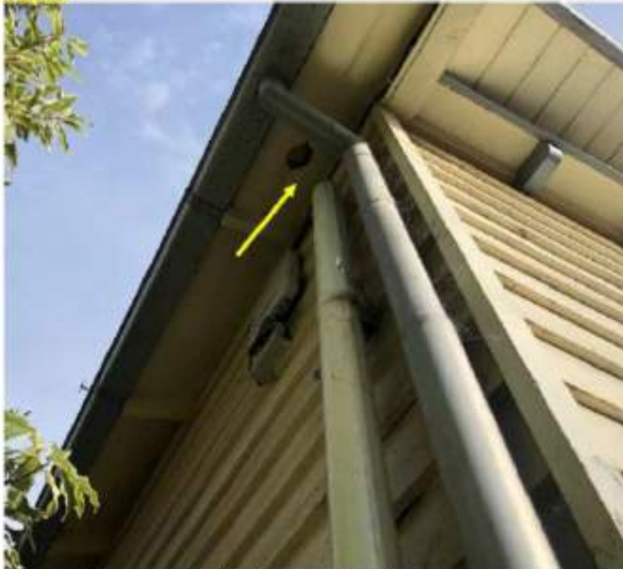
Disconnected storm water pipe
