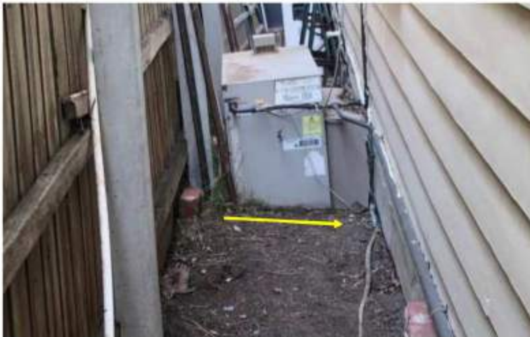
Soil profile graded towards subfloor
