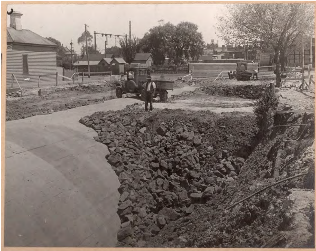
Figure 7: View of the western end of Bunbury Street, 1927-1928, during the addition of basalt fill around the newly constructed tunnel. The steps of the pedestrian overpass from the railway station are visible at top right of frame. (Source: SLV).
