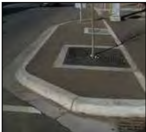
SF 012 Pavement Sawn bluestone kerb extension spoon drain
