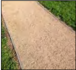
OS 001 Footpath Granitic Gravel with Timber Edge
