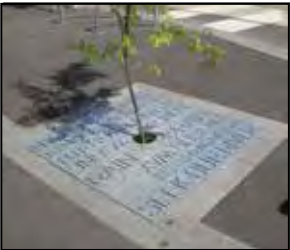
SF 601 WSUD Tree Pit Kerb entry water inlet with laser cut tree grate
