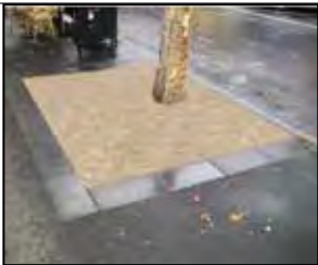
SF 601 WSUD Tree Pit Kerb entry water inlet with laser cut tree grate
