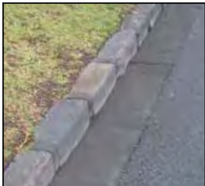
SF 007 Kerb Bluestone pitch kerb and coloured concrete channel
