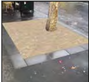
SF 603 Tree Planting Bay Granitic gravel with bluestone edging
