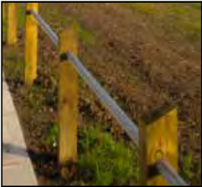
OS 501 Boundary Treatment Cypress Pine Posts and Galvanised Rail
