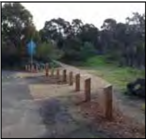
OS 501 Boundary Treatment Cypress Pine Posts and Galvanised Rail
