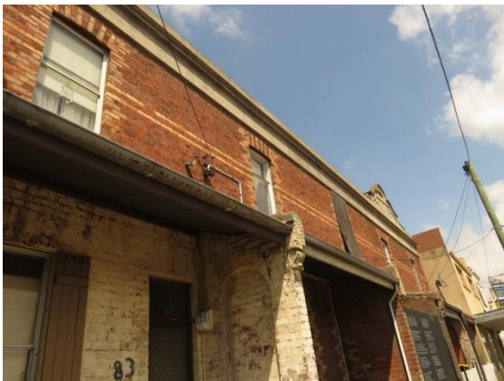
Figure 3 better preserved part of upper level (83-87) with cemented parapet cornice, raised entablature, cream brick string moulds.
