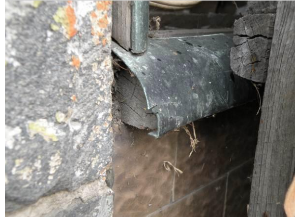
Above: 20 th century metal capping on timber window frames of shop front.
