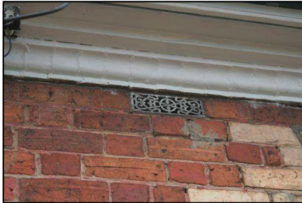
Figure 7 cast-iron 'air brick' and terracotta eaves moulding
