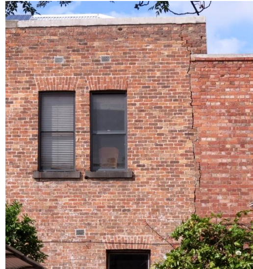
Figure 29 Cavity brick wall for house, upper level windows and stone sills on boundary, English bond for earlier bakery.
