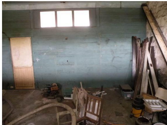
Above: Internal timber stud wall (to back room).
