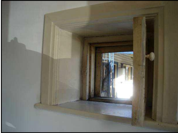
Figure 10 Timber reveals of south window (COM)
