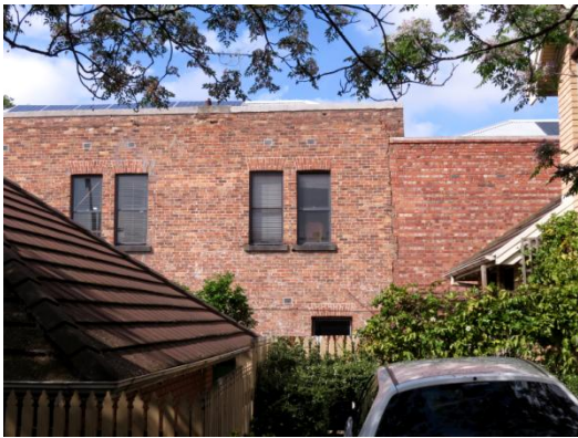
Figure 35 North wall of house and bakery showing the staged development
