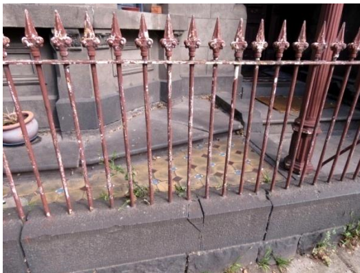
Figure 31 Fence, paving detail showing dressed basalt and tiles.
