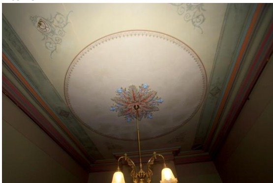
Figure 67 Ceiling south-west originally main room of house, 2012: painted cast plaster central flower, encircled with a stencilled frieze border and lyre patterns in the 4 corners, with lozenge patterns in the main border
