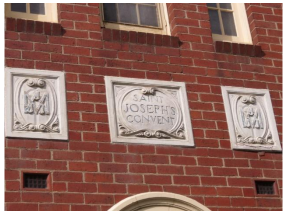
Figure 75 Pressed cement detailing
