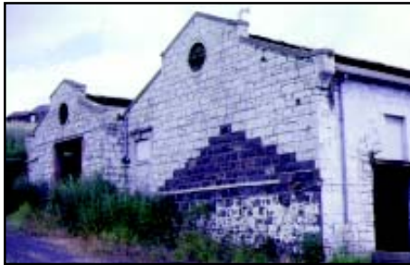
Former Melbourne Meat Preserving Works, Footscray. Source: Heritage Victoria.
