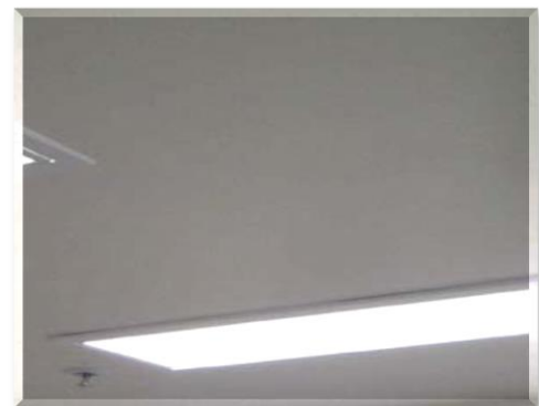
RECESSED LIGHTS WITH SHATTERPROOF COVER
