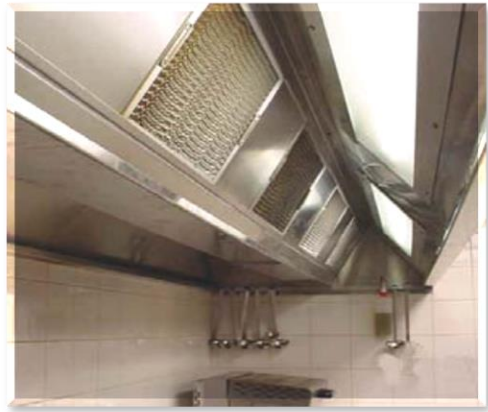
COMMERCIAL MECHANICAL EXHAUST SYSTEM ABOVE ALL WORKING APPLIANCES
