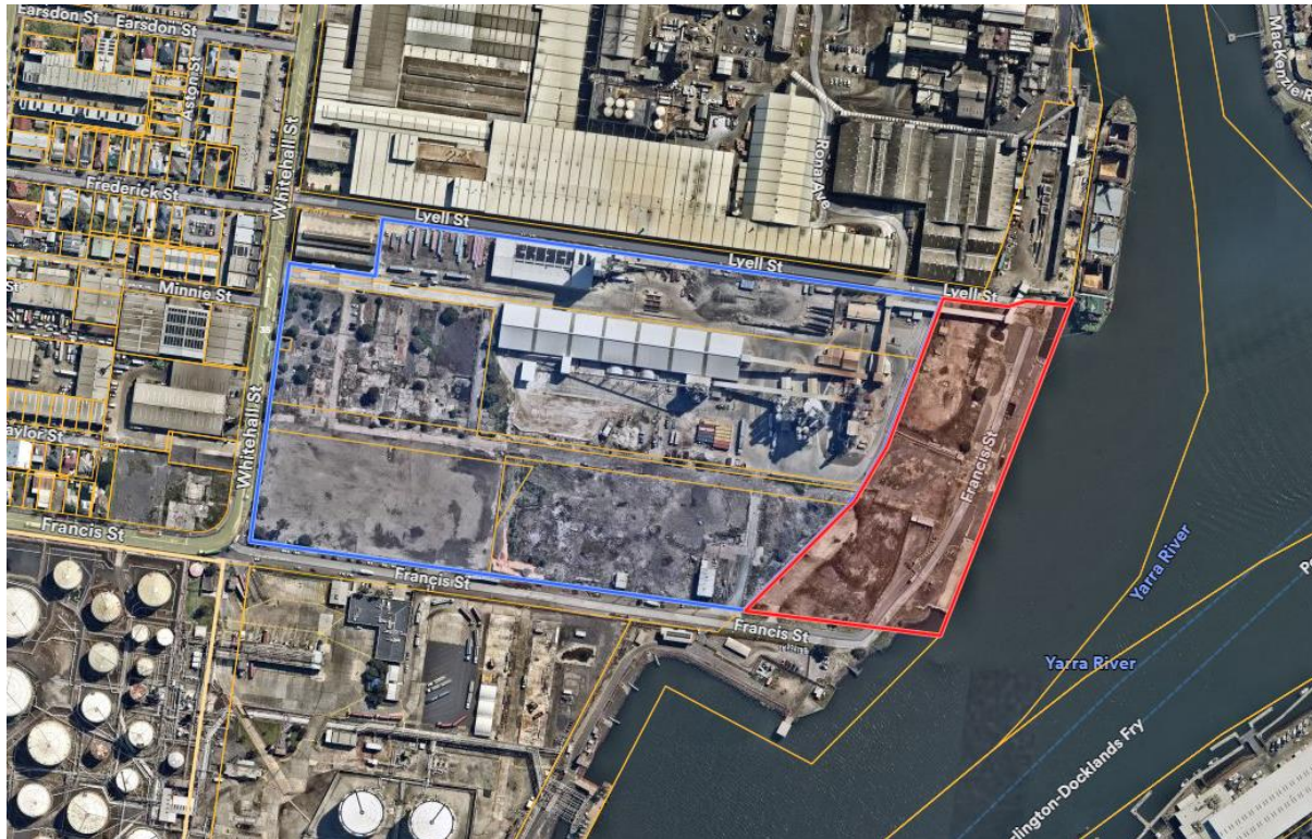
Figure 2: The subject site in blue and adjoining Port Zone land shown in Red. Source: Nearmap 2024.
