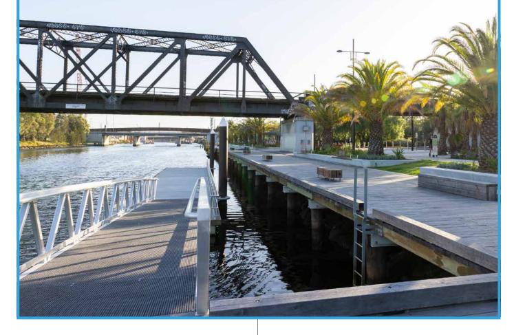
COUNCIL IS PROPOSING FURTHER UPGRADES TO FACILITIES AND AMENITIES ALONG THE MARIBYRNONG RIVER WATERFRONT TO COMPLEMENT THE COMPLETION IN 2022 OF A NEW 230-METRE-LONG TIMBER BOARDWALK WITH A FIXED LOWER LANDING AND FLOATING PONTOON AT FOOTSCRAY WHARF.
