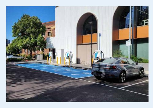
A new publicly available electric vehicle (EV) charging hub has been installed at the Civic Precinct and Community Hub in Footscray, featuring three dual DC chargers. Each charger delivers up to 150kW of power, enabling up to six electric vehicles to charge at once.
