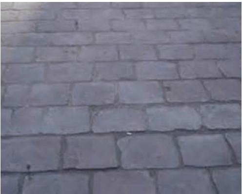
Sawn bluestone pitcher at raised transition thresholds
