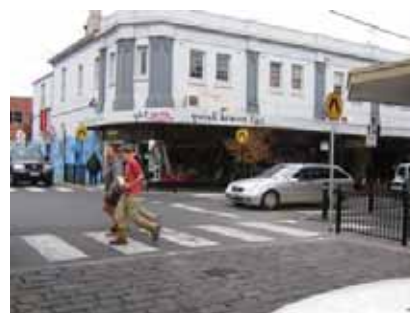
Similar raised pavement treatment in Prahan. Road is raised flush with kerb.
