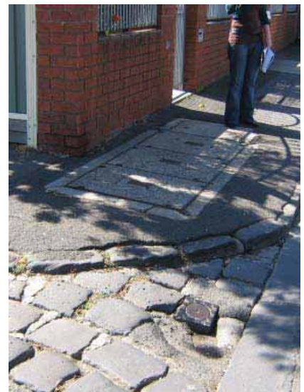
Wood Street/Murray Street intersection. Uneven and cracked footpath creates tripping hazard.
