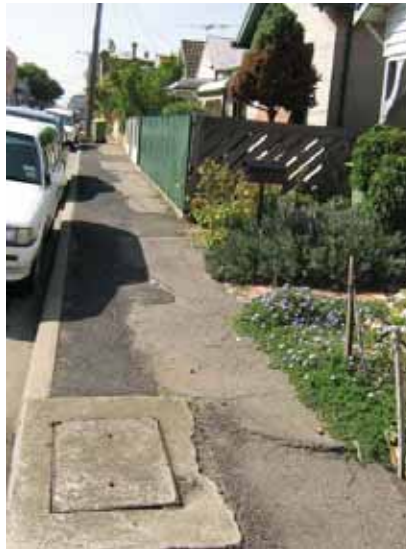
Simpson Street, footpath cracked, patched and generally in poor condition.
