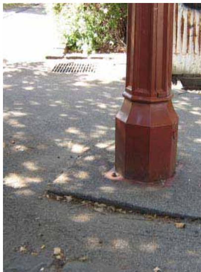
Light pole footing creates potential trip hazard in park (off Anderson Street).
