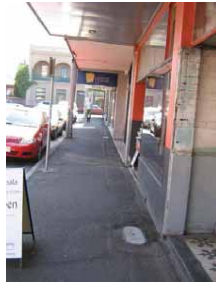
Ballarat Street, Telstra trench reinstatement uneven and unsightly.
