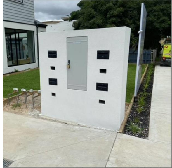
Image 2 – high structure in front setback ✗ Unacceptable location for electrical meterbox
