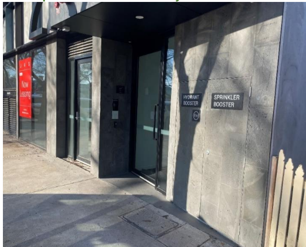
Image 3 - integrated into side wall of development ✓ Acceptable location for fire hydrant/booster
