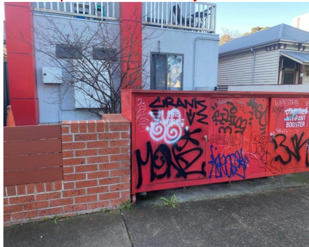
Image 4 – standalone structure in front setback ✗ Unacceptable location for fire hydrant/booster
