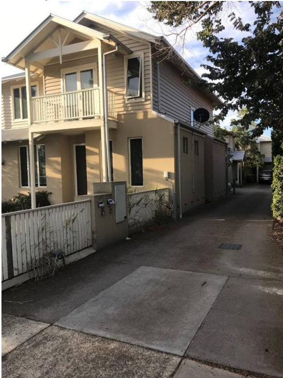
Image 3 – setback and integrated into fence ✓ Acceptable location for electrical meterbox
