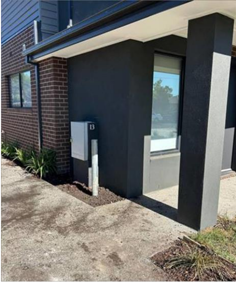
Image 1 – integrated into side wall of development ✓ Acceptable location for electrical meterbox
