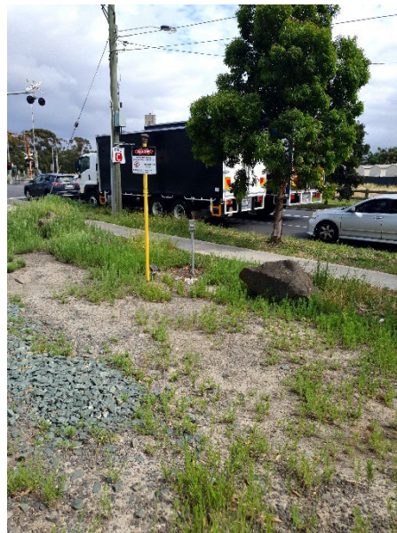
Figure 6-2 Pipe line markers
