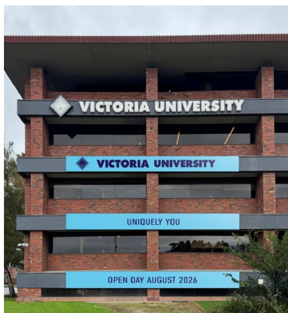
Figure 9 Building K – East Elevation Signage
