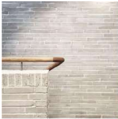
New ground level wall cladding
