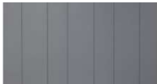
New first floor wall cladding
