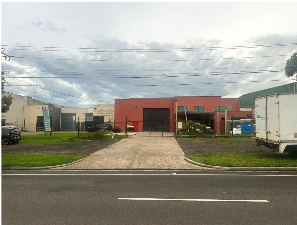
FIGURE 2: SUBJECT SITE (SOURCE: SITE INSPECTION)
