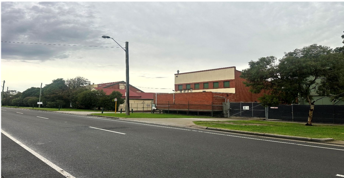
FIGURE 6: CRANWELL STREET (SOURCE: SITE INSPECTION)
