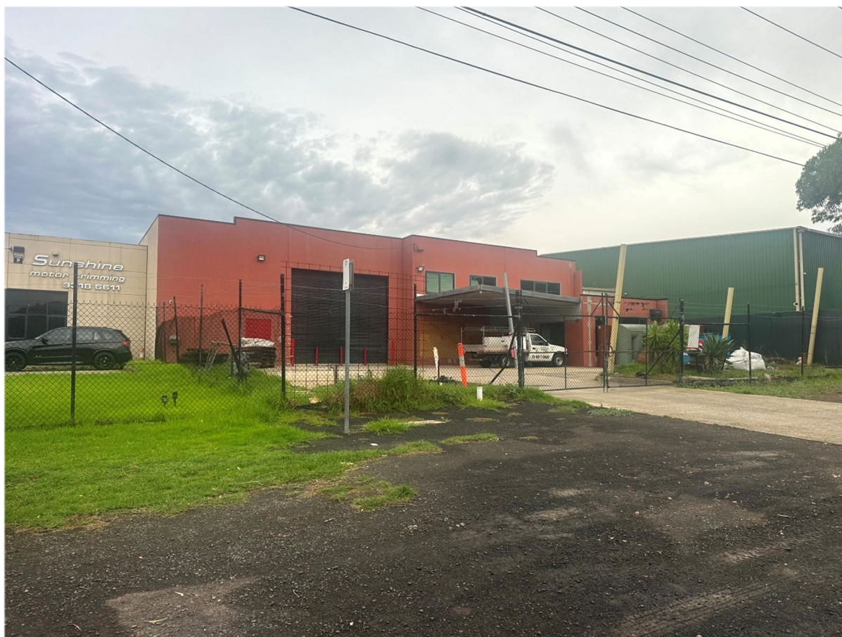
FIGURE 3: SUBJECT SITE (SOURCE: SITE INSPECTION)
