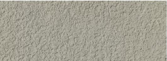
PORCH RENDER: RENDER AS PER ORIGINAL PAINTED DULUX POWDERED ROCK
