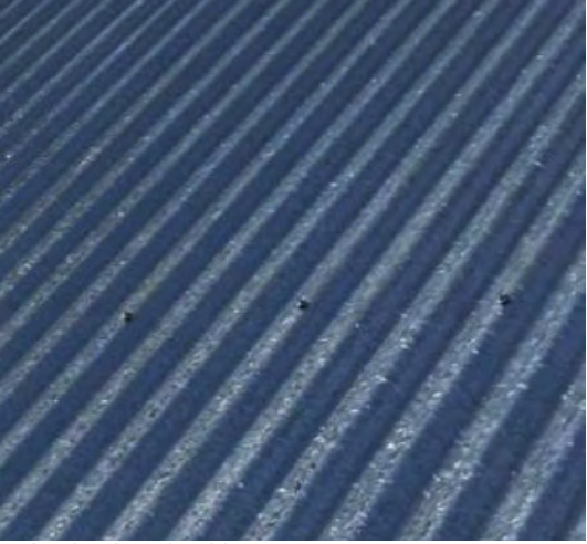
EXISTING RESIDENCE ROOF: CUSTOM ORB GALVANISED ROOF SHEETING HERITAGE GRADE Z600
