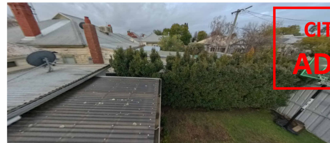
REAR YARD LOOKING EAST
