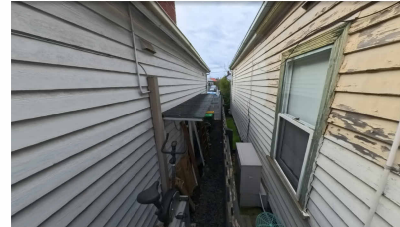
EAST SIDE LOOKING NORTH
