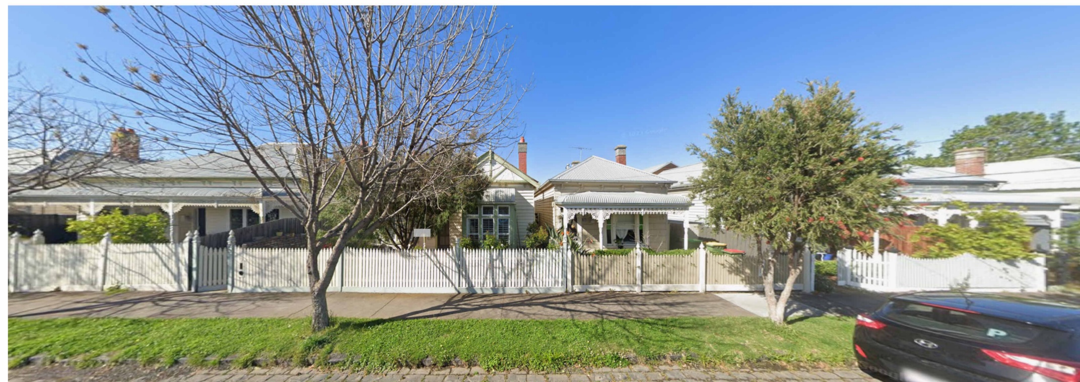
No 21A BROWNING STREET, SEDDON
