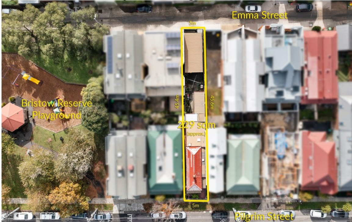
Figure 3: Aerial Photo of subject site 124 Pilgrim Street Seddon.
