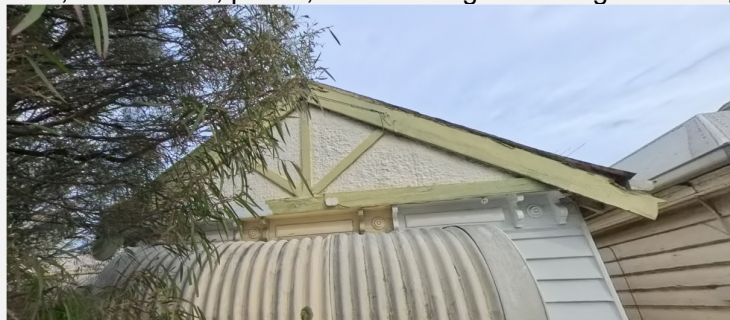
Image of existing gable weathering
