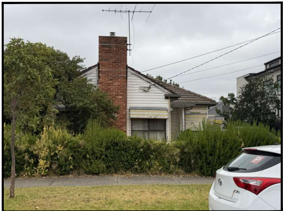
No.37 FISHER STREET ADJOINING NEIGHBOUR (TO THE RIGHT)
