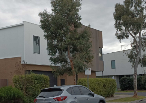
Point A. 7 Beame Street - Recent 1F Addition
