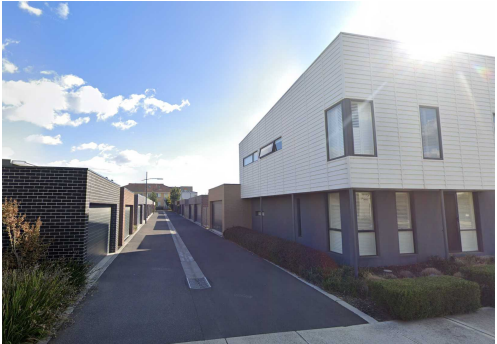
Point E: View into the laneway toward the subject site
