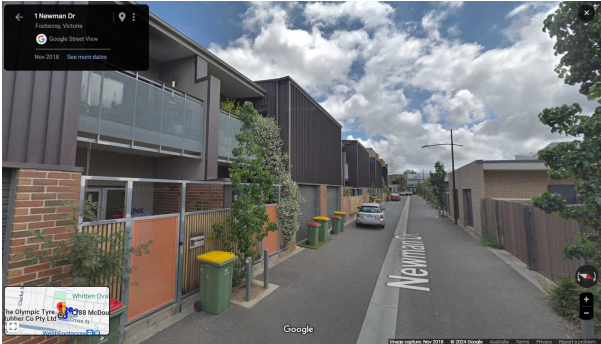
Point C. Rear of Olymic Tyres Building - Newman Drive
