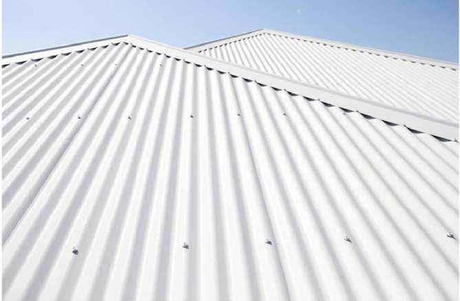
RF01 - CORRUGATED METAL ROOFING - COLORBOND SURFMIST
