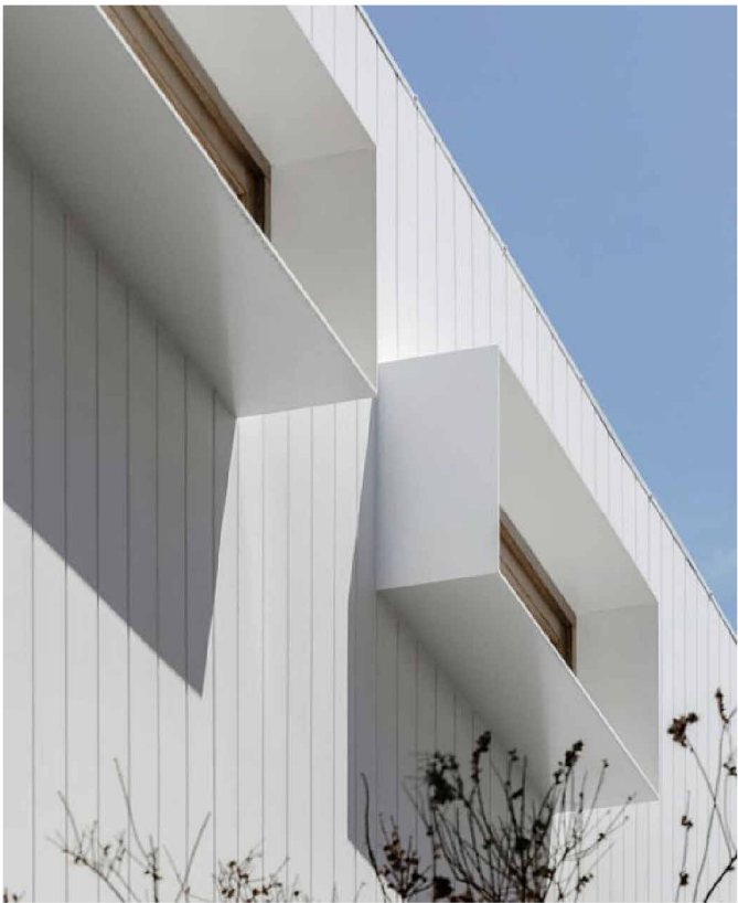
MC01 - METAL CLADDING - SURFMIST PC02 - WINDOW SHROUD & SUNSHADE - POWDERCOATED EVENING HAZE
