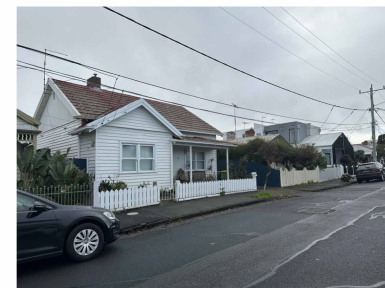
STREET VIEW 3 - TOWARDS EAST
