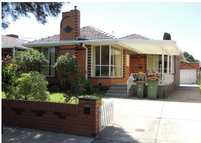
25 Creswick St, one of the group of houses on the site of the Laughton's Iron foundry showing dichromatic brickwork, hipped terracotta tiled roof, prominent chimney with "Waterfall" top, steel windows including corner windows, decorative wrought iron balustrade and driveway gate, matching brick fence and garage. Source, M. Kenna 2020
