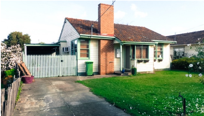
Housing Commission of Victoria weatherboard bungalow at 81 Wellington Street, circa early 1950s. It has a glazed terracotta tile roof, prominent red brick chimney, timber-framed, sash corner windows and porch under sloping front roof. Others in the street have slight variations on the design. Source, M. Summerton, 2020
