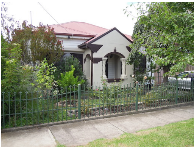
9 Dempster Street, West Footscray. One of a small number of houses in Dempster Street with 'Conite' façade. This example also has Spanish Mission influenced details such as barley sugar columns and arched openings to the porch. Source, M. Kenna 2020
