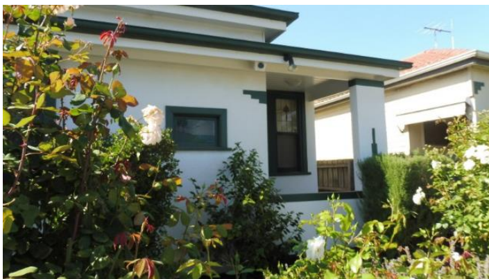
Numbers 1A and 2A Nesnah Street are atypical of houses in the Hansen Estate. They were built on narrower allotments at the end of the dead-end street, with no provision for side drives. The freestanding pair share basic, functional forms with conite facades, small enclosed porches, and windows with decorative lead lighting. 1A retains its original roof of metal, simulated terracotta tile sheeting. Source, M. Summerton, 2020
