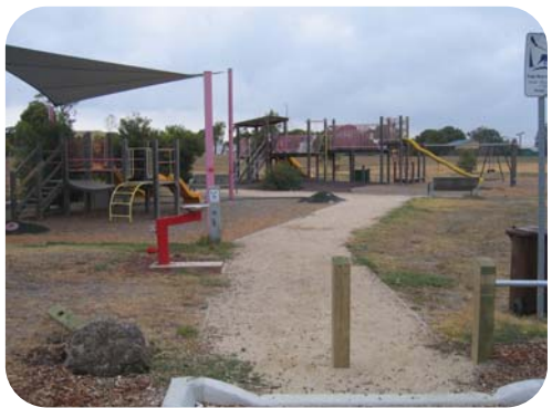
Playground, entry from Robert Street carpark
